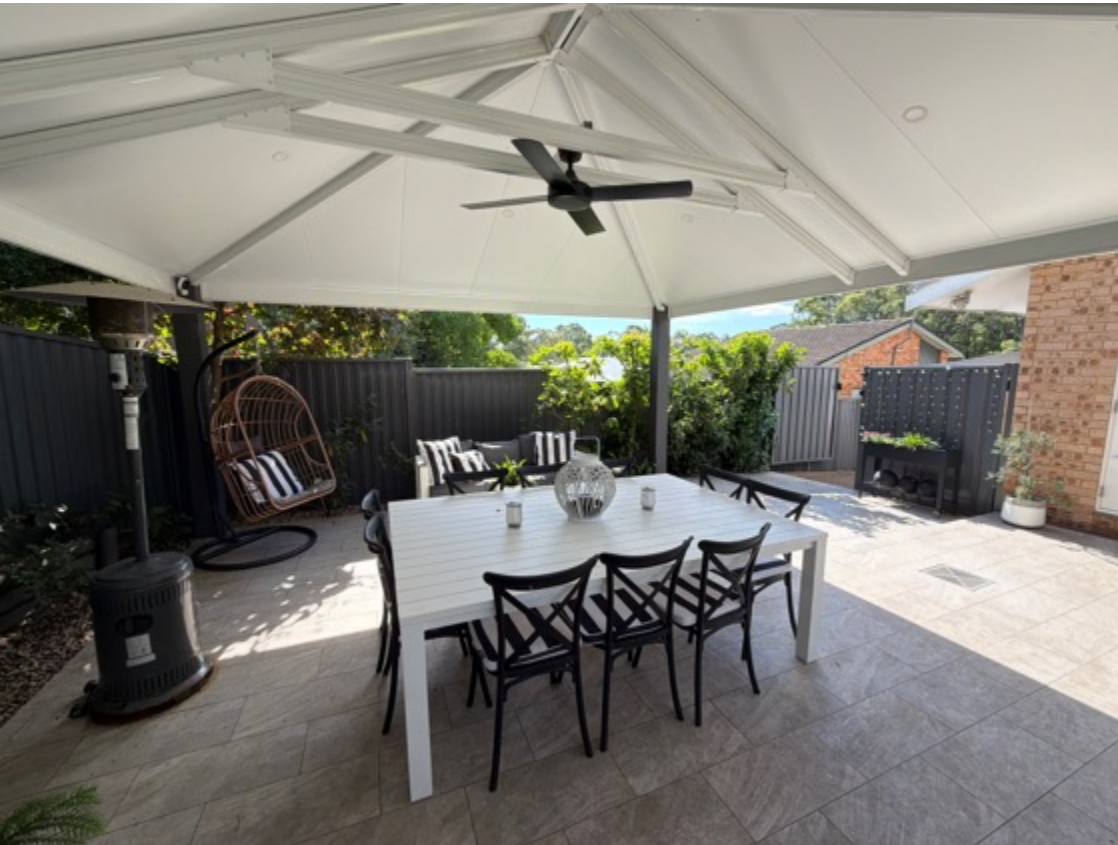
The rear pergola checked is structurally sound.
