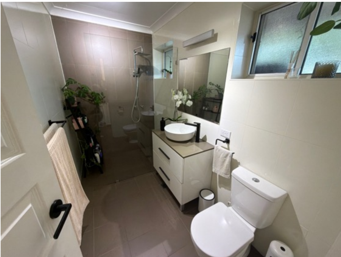
Common bathroom water services tested, functioned at the time of inspection.
