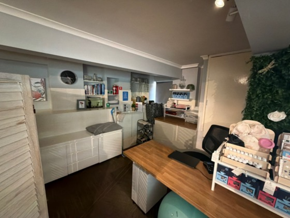
The kitchenette is in serviceable condition.
