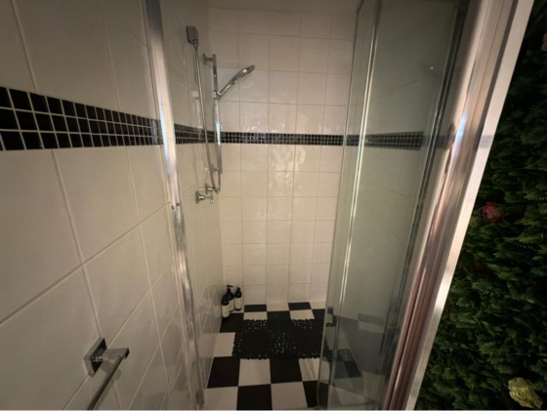
Water pressure tested, is sufficient.
