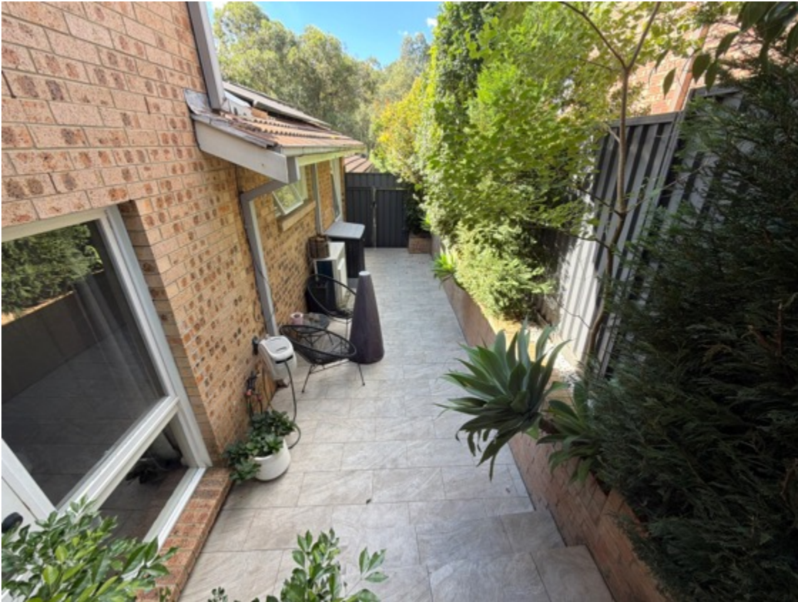
Site fences are in serviceable condition, isolated sections have minor dents and are leaning (consistent with age.)
