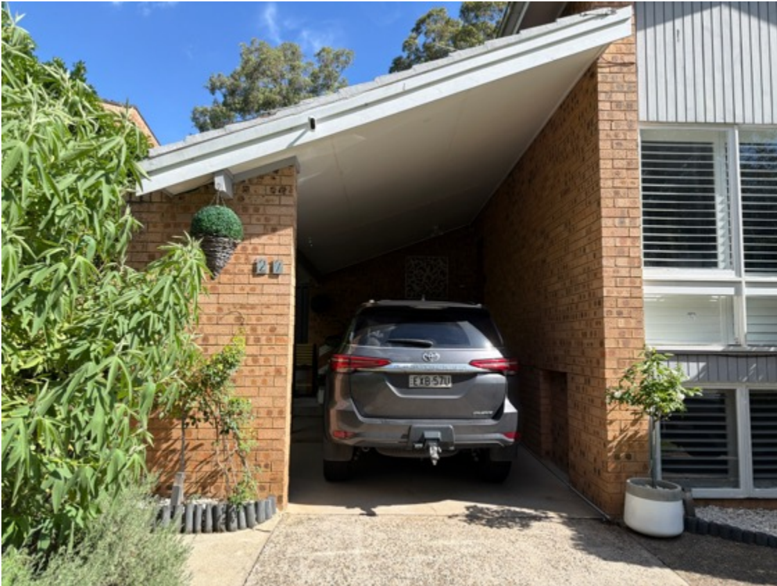
The carport checked is structurally sound.
