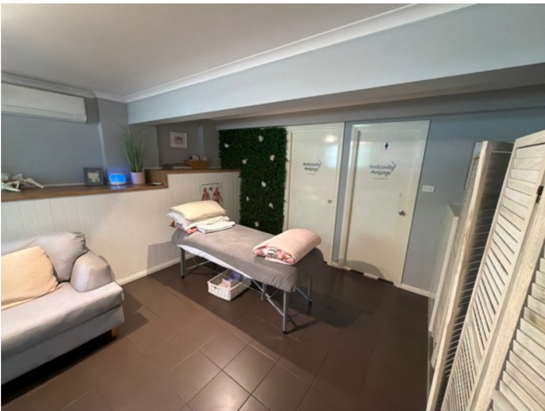
Lights tested, functioned at the time of inspection.
