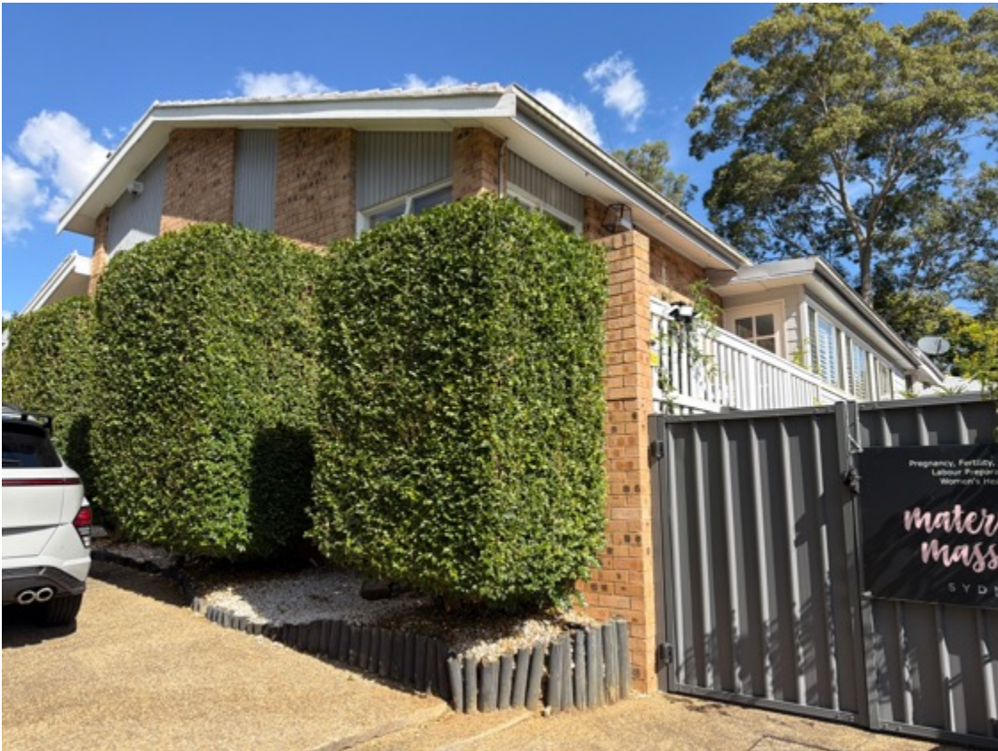
Exterior windows and doors present in satisfactory condition for the age.
